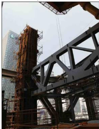
Fig 2: Outrigger Truss Connected to Perimeter Columns
